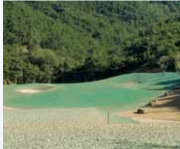
Golf Course Construction
